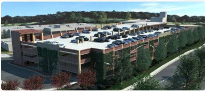
New Parking Structure at Henry Mayo Newhall Memorial Hospital
